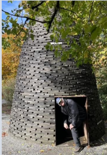
Night Blooming (Taiji Miyasaka & David Drake) is a catenary dome constructed using lumber salvaged from grain elevators in the Palouse region of Eastern Washington. The patterns of voids provide subtle changes of light and shadow.
